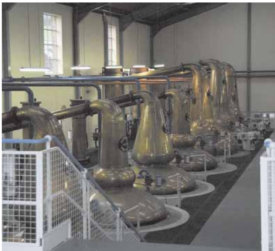
Reporting and control of tank levels, temperature and flow rates are just some of the applications the GT1020 HMI can be used for.
